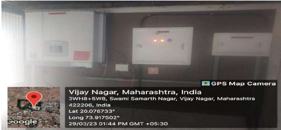
Installed Solar Charge controller
