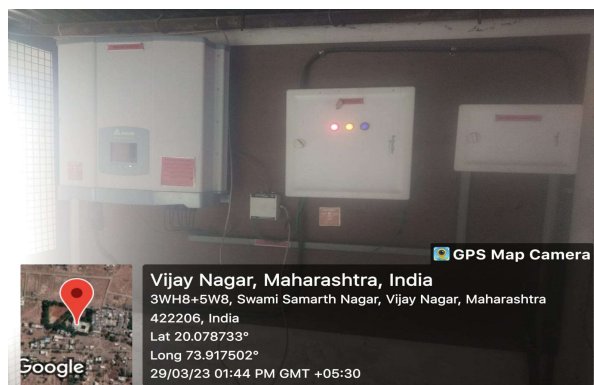
Figure 15. Installed Solar Charge controller
