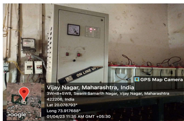
Figure 17. On-line UPS with Battery
