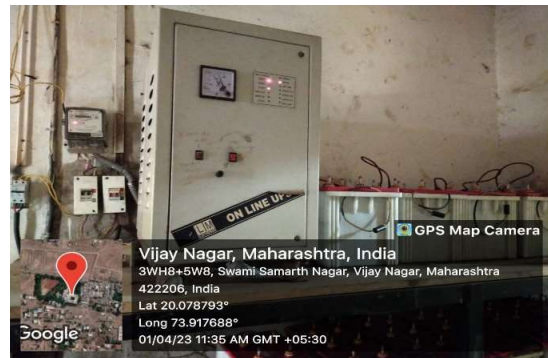
Figure 17. On-line UPS with Battery
