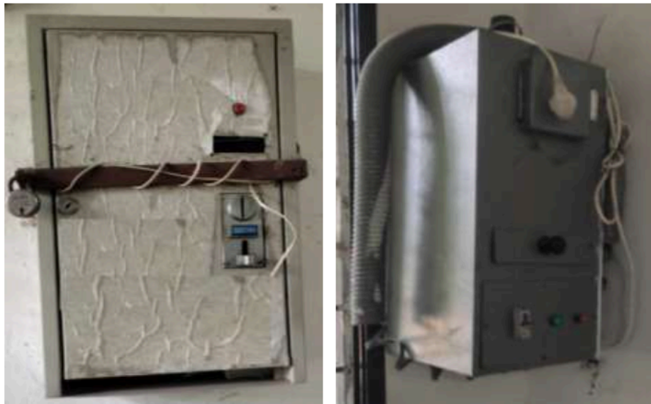
Photo No. 21 Sanitary Pad Vending Machine Installed in Girl's Rooms
